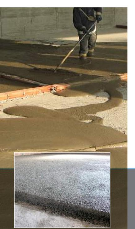
**iSCREE 24** are synthetic polypropylene fibres specifically designed for screeds reinforcements:
